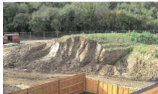
Long term stockpile of stripped topsoil left with only weed vegetation
