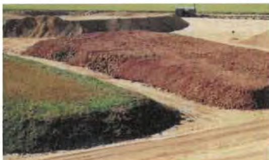
Clearly defined stockpiling of different soil materials
