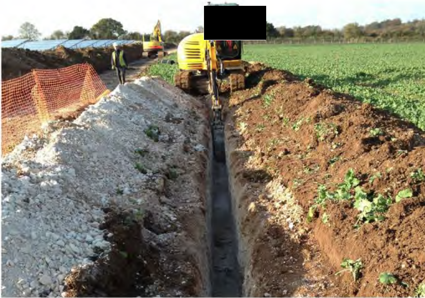
Cable trenching, showing topsoil stripped and set to one side, with subsoil placed on the other side ready for reinstatement (photo courtesy of British Solar Renewables)
