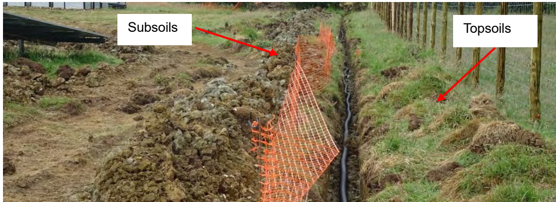
Insert 43: Subsoils Dug out of the Trench
