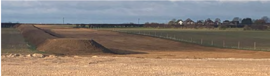
Insert 46: Example of temporary bund (example shown in a water pipeline)
