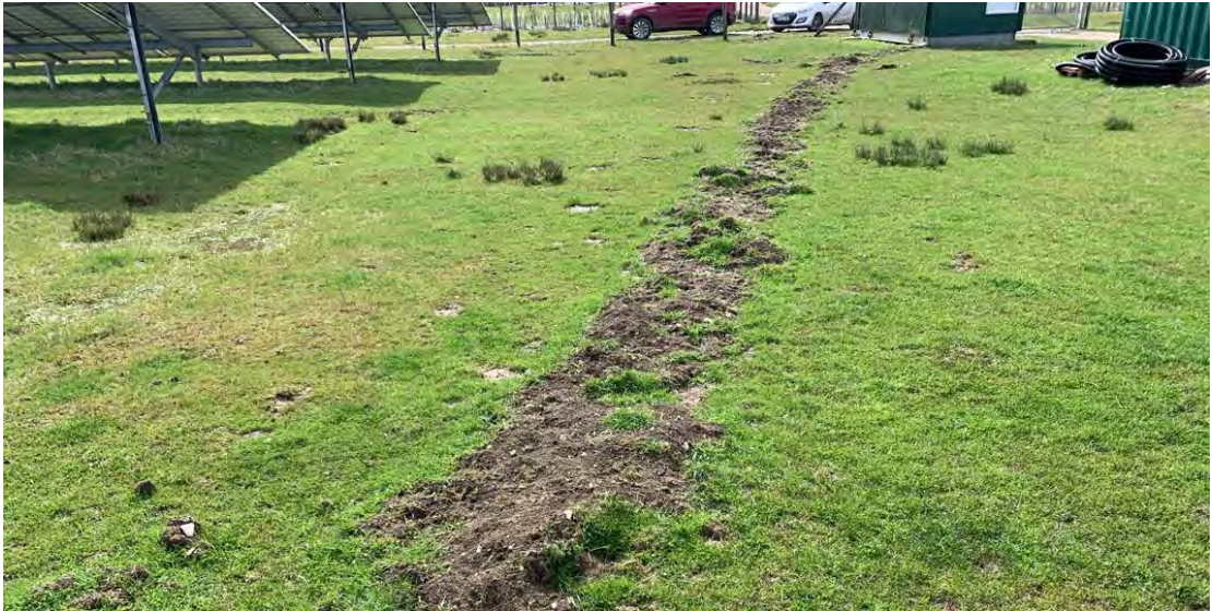
Insert 56: Trench During Wet Period
